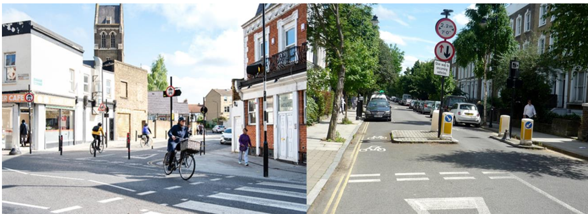
Wordsworth Road filter at junction to support the provision of a signed cycle route (left) and road narrowing to facilitate traffic calming (right)
